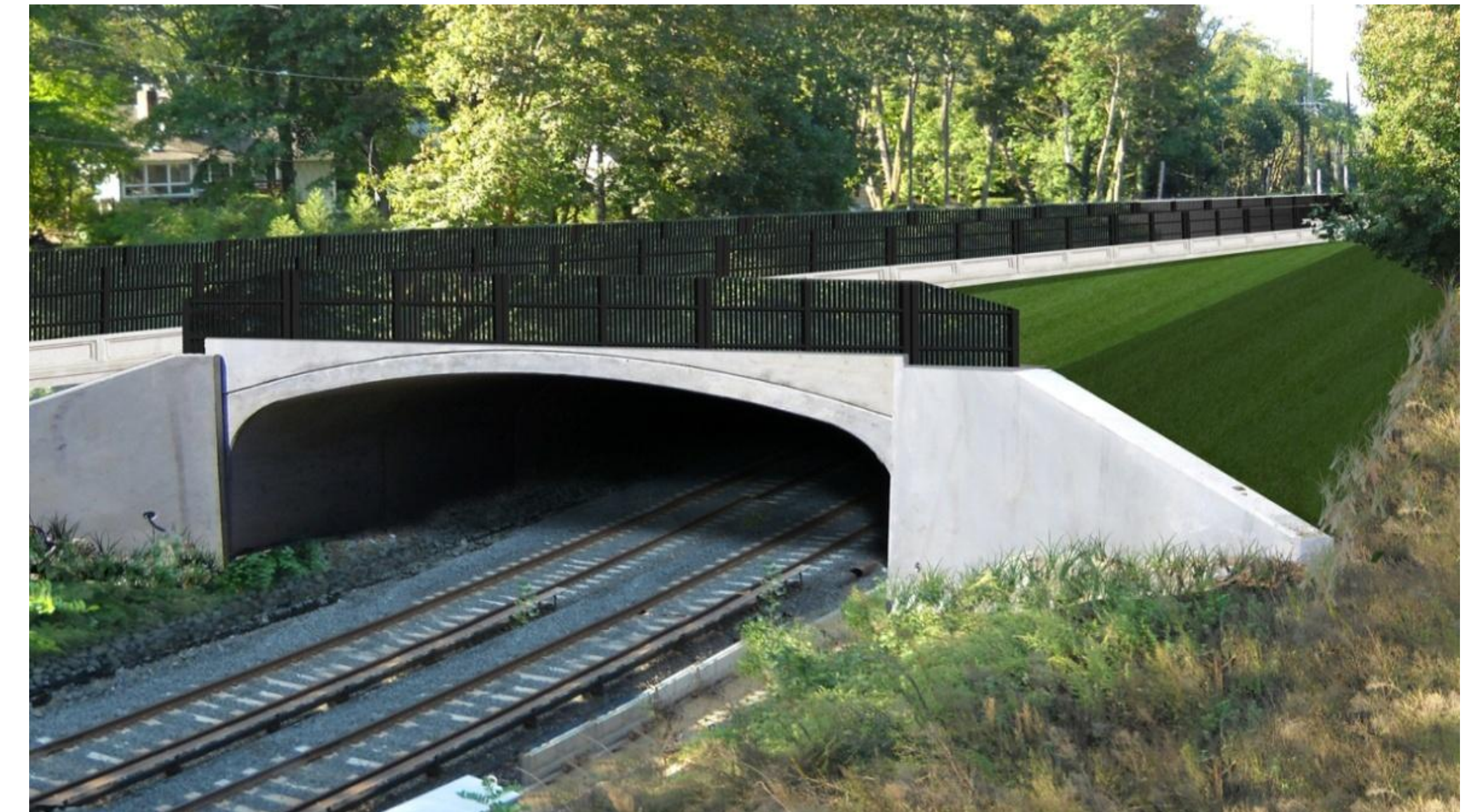
Proposed Pre-Cast Concrete Arch System Looking West
