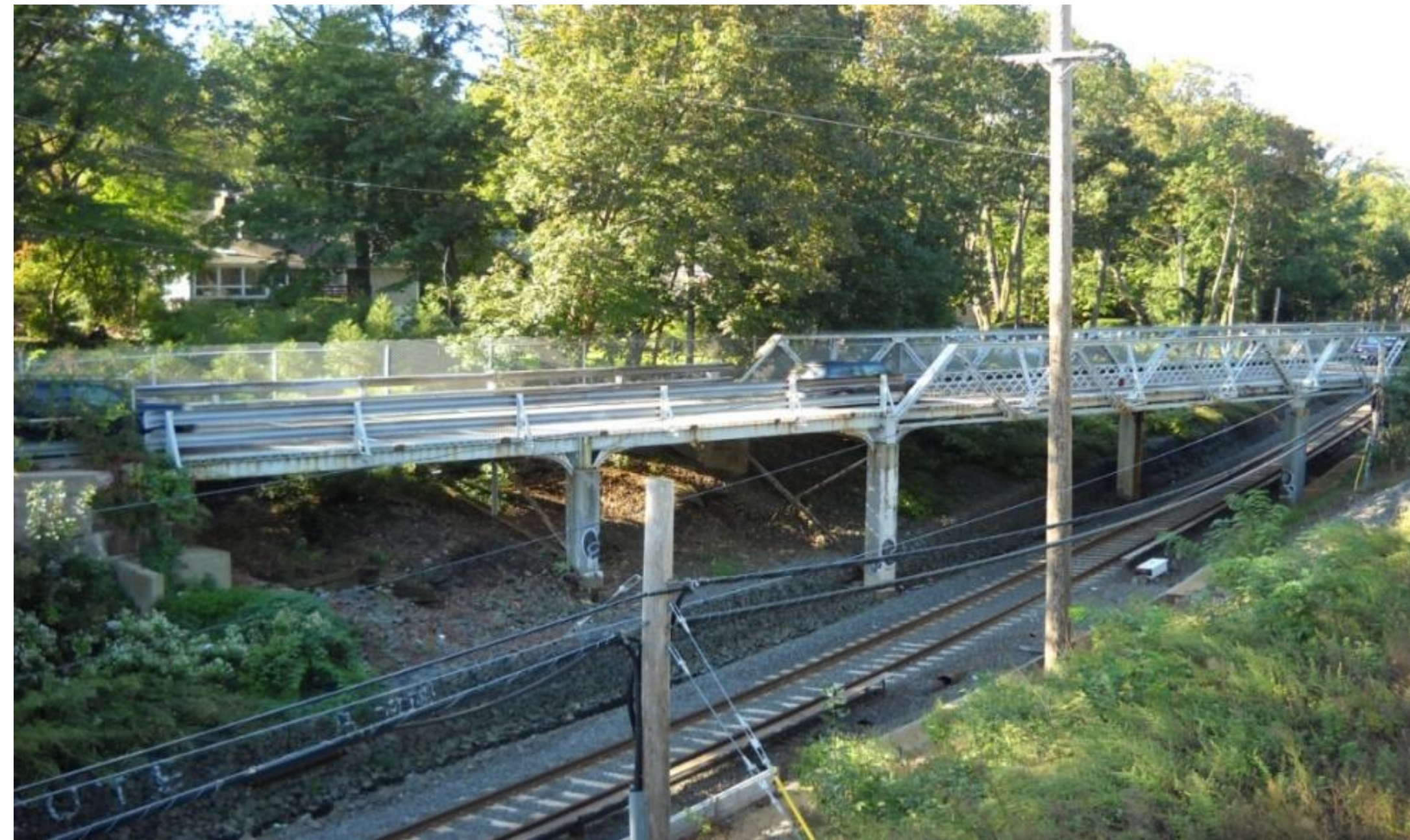
Existing Colonial Road Bridge Looking West
