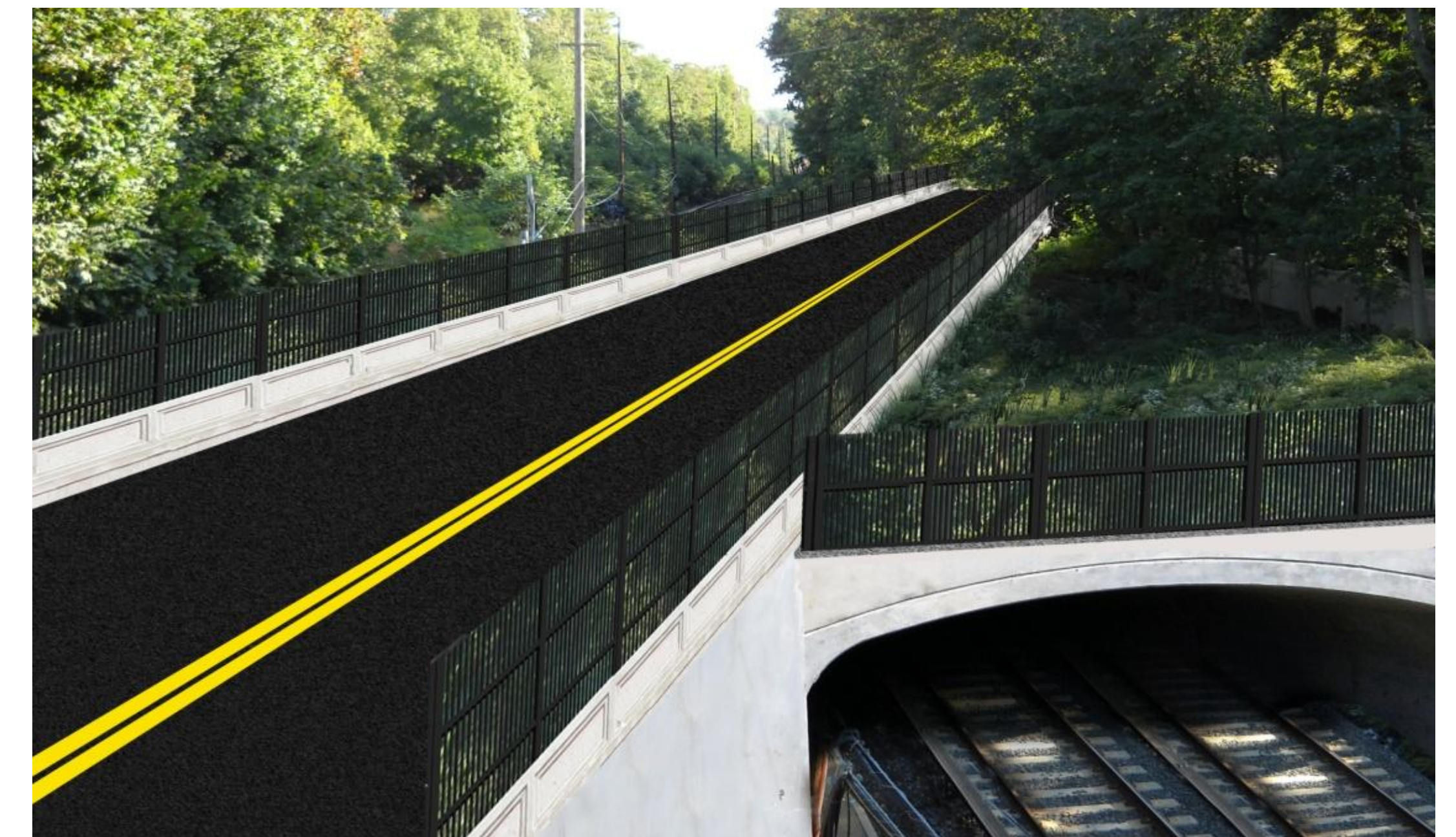
Proposed Pre-Cast Concrete Arch System Looking East
