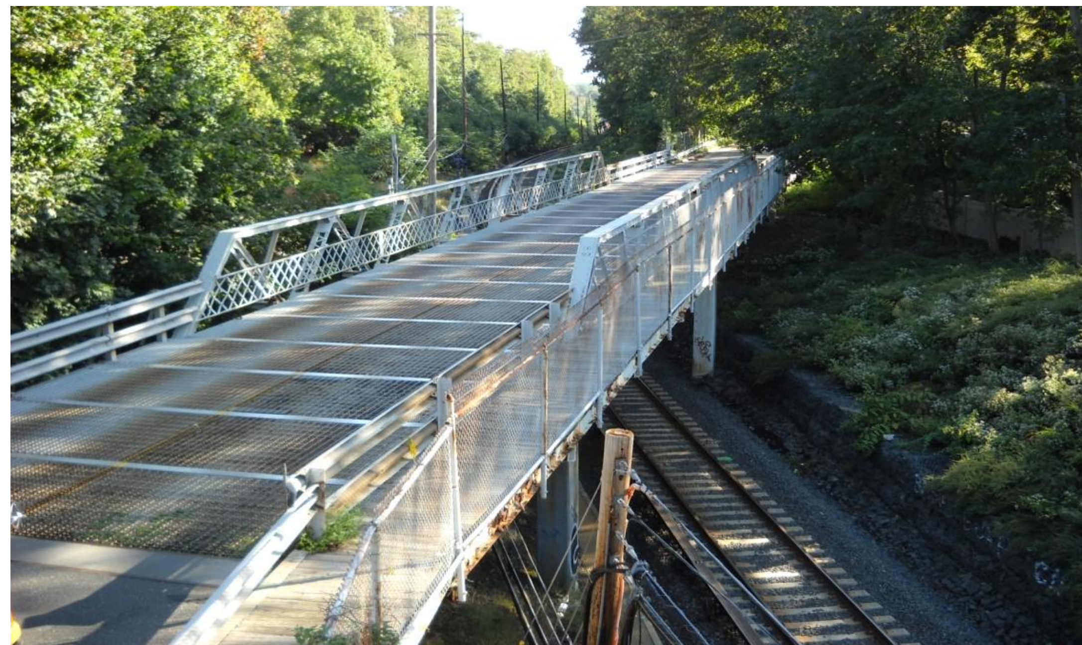
Existing Colonial Road Bridge Looking East
