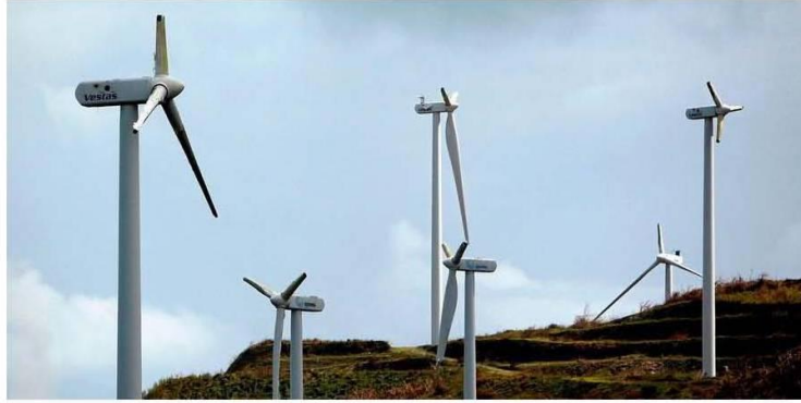
Onshore wind turbines in Puerto Rico damaged by Hurricane Maria in 2017. Photo: AFP/Getty
