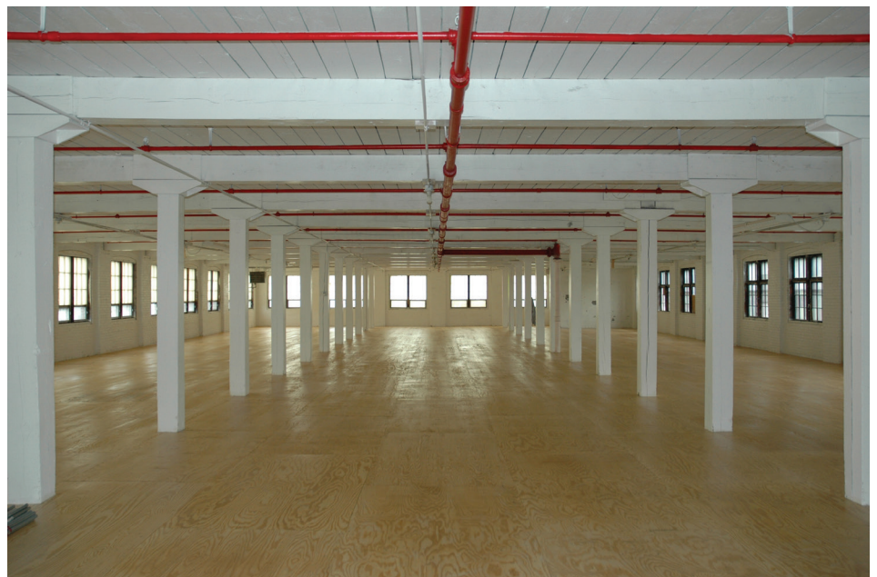
Floor space ready for a manufacturer at HARC Business Park. (Photo courtesy of Herkimer ARC)
