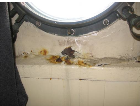
Hole in bulkhead under porthole
