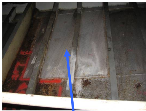
Replaced plate in shell
