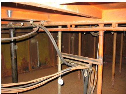
Void space under wheelhouse
