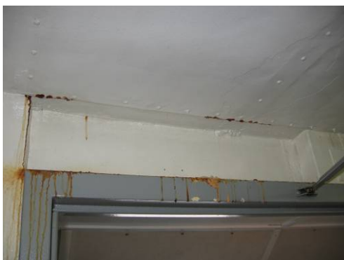
Leak from boat deck
