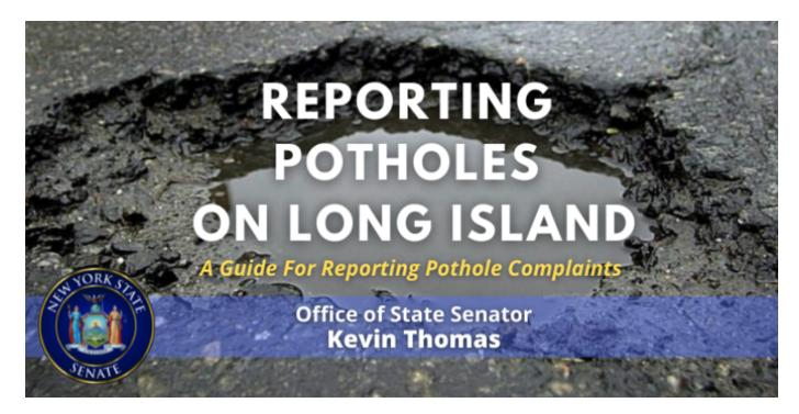
Spring temperatures warm the cold pavement, melting and evaporating any ice. This creates air pockets that can eventually cause the pavement to break up. A winter of heavy snow or rain and several freeze-thaw cycles can mean a big pothole season ahead.
