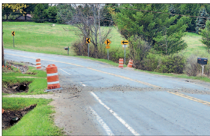
Drainage pipes being replaced on Powderhouse Road in Corning last spring.
